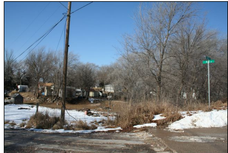
Photo 3: Absence of sidewalks fails to meet ADA standards
