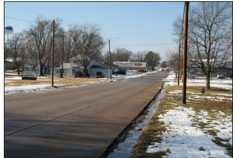
Photo 6: The absence of a sidewalk network fails to meet ADA standards
