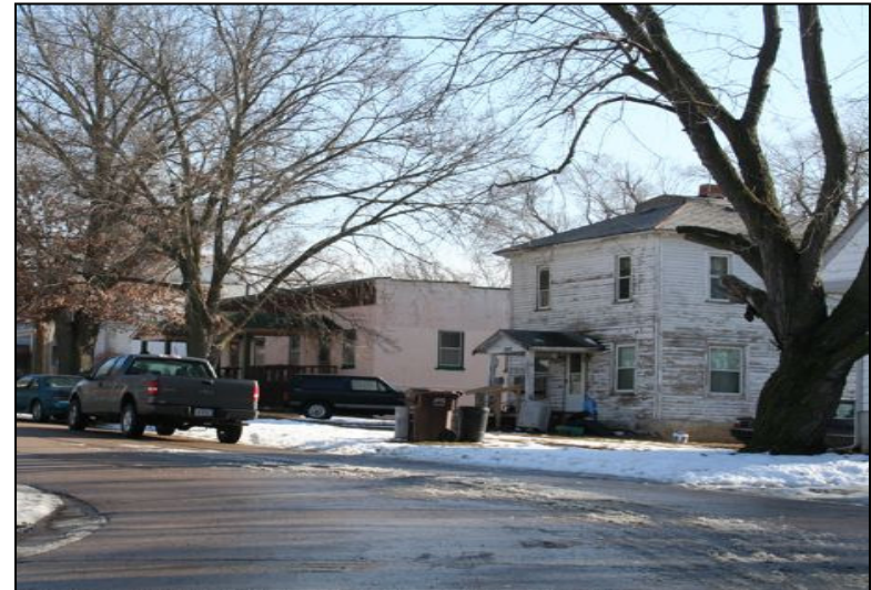
Photo 4: Aged and dilapidated buildings provide evidence for substandard determination
