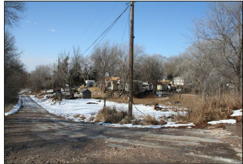
Photo 1: Deteriorating structures and roadways
