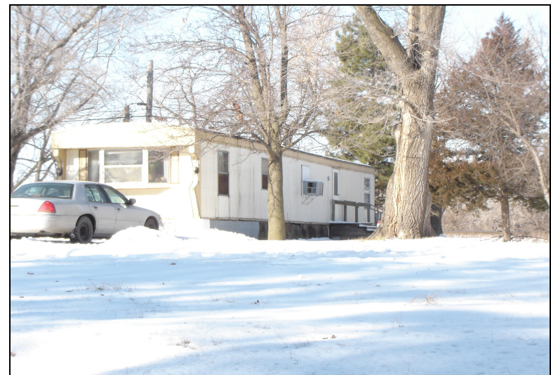
Photo 9: Many structures located along Highway 6 do not comply with the City of Ashland Zoning Ordinance
