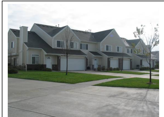
Example of Single-Family Attached
